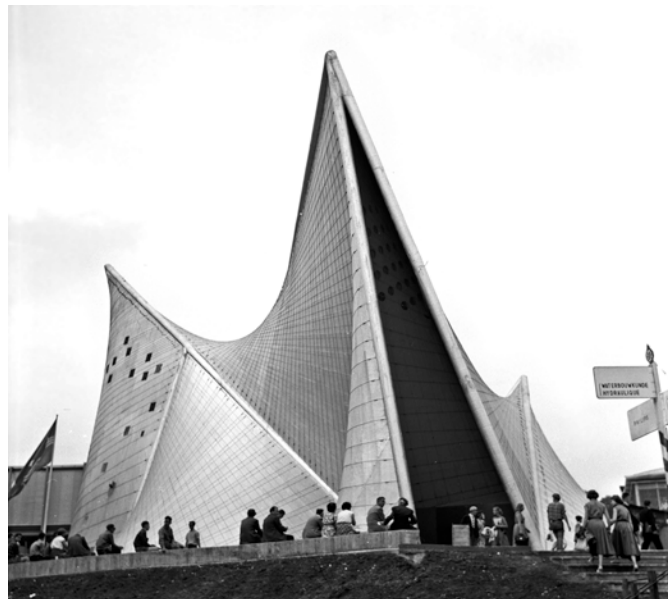
Figure 7. Architectural fulfillment of the musical project: Philips Pavilion (1958).
