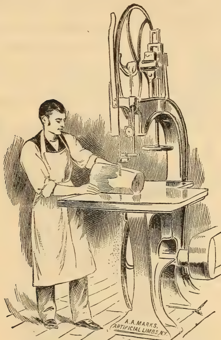
No. 1191.—BAND SAW AT FACTORY.
